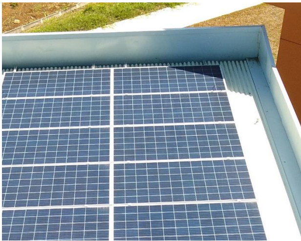
Fig. 1. Example of a solar panel with a partial shadow.
